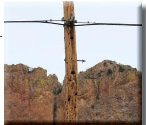
**Notice the woodpecker holes. This is one of the two poles recently replaced in Big Bend National Park using a helicopter. It also had bear damage at the lower end of the pole.**
