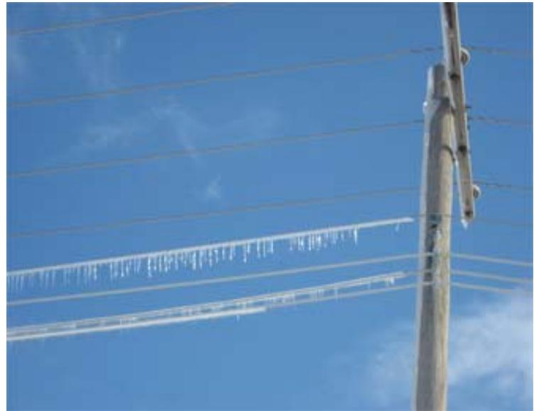
Each square inch of ice weighed approximately 2 ounces. That may not seem like much, but an average line span of 300 ft., or 3,600 inches from pole to pole, with a one inch accumulation of ice would weigh an additional 432 pounds per span. A three-inch accumulation of ice would weigh an additional 1,296 lbs. per line span.
