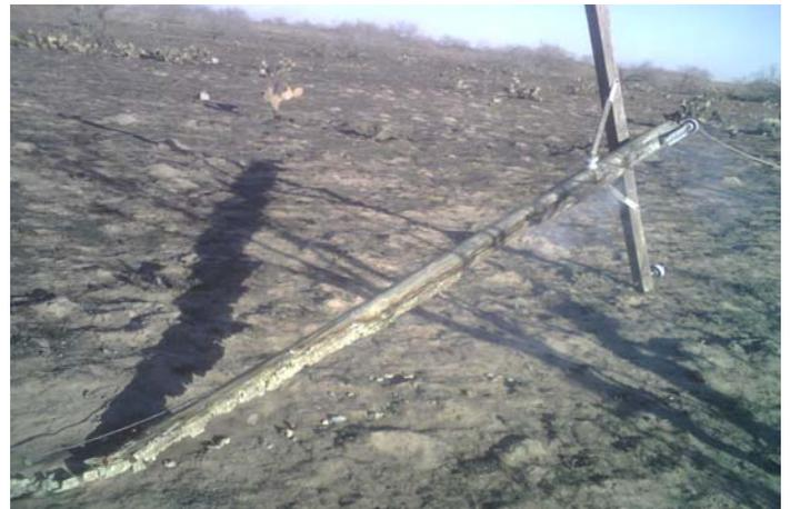
Wildfires caused substantial damage to RGECs poles and equipment last year. The Fort Stockton and Carrizo Springs areas were particularly hard hit, losing over 90 poles to fires between the first of the year and mid-May alone.
