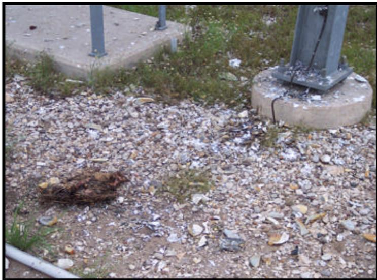
**A “fried” owl caused a massive power outage and equipment damage at the Brackettville substation in May. (Notice the ashes and melted metal.)**
